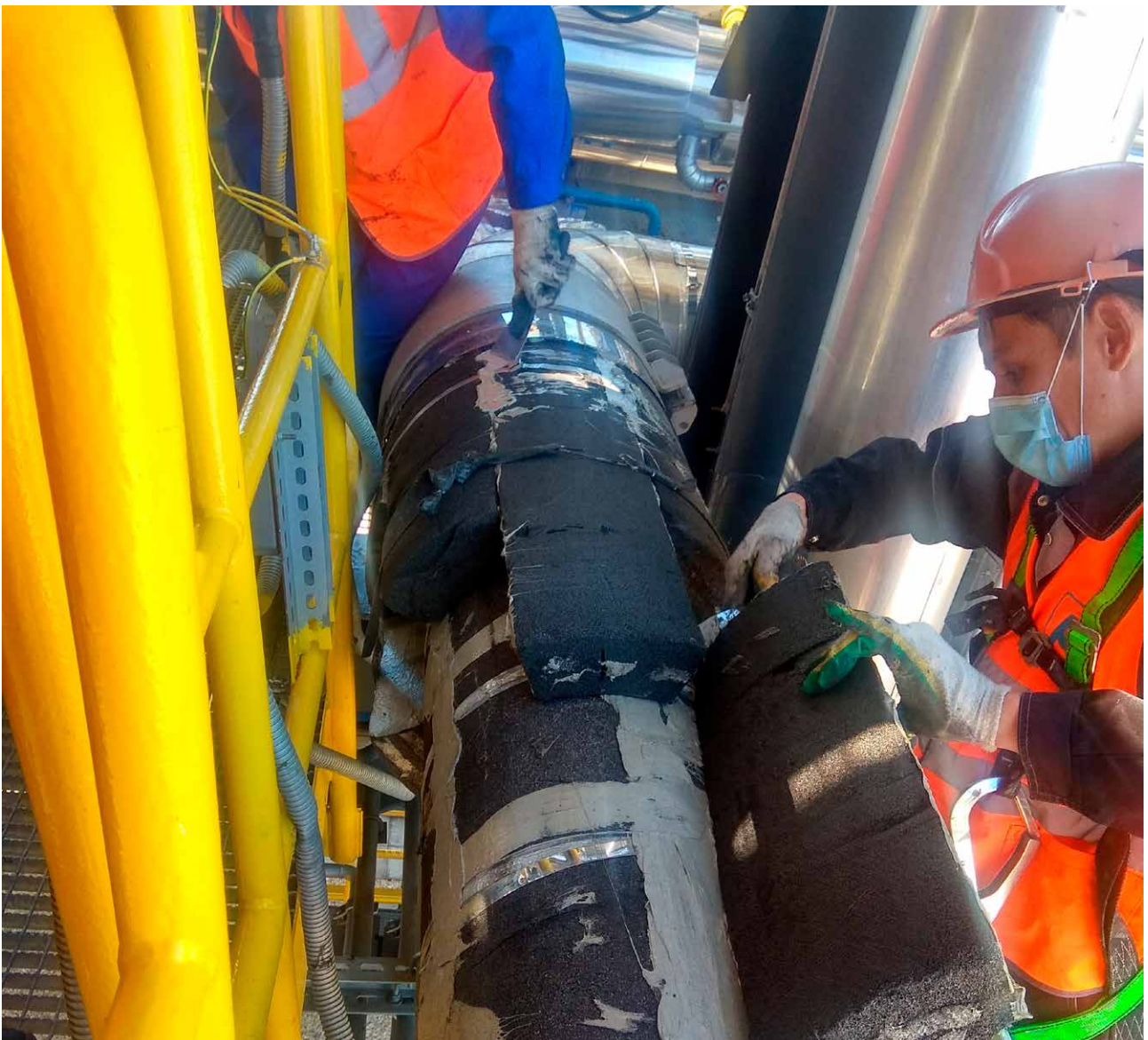
Insulation work in Russia
